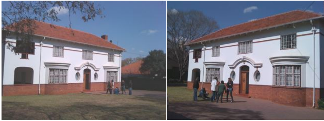
The office building of HRDI, where the training programmes take place. The building accommodates a group of 10 to 20 persons during the training programme.
